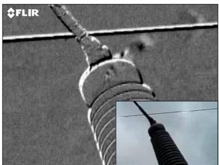
SF<sub>6</sub> leaking from the bushing of a gas circuit breaker
