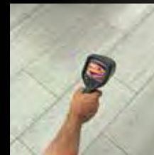
Check floorheating for leaks
