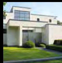
Find insulation problems
